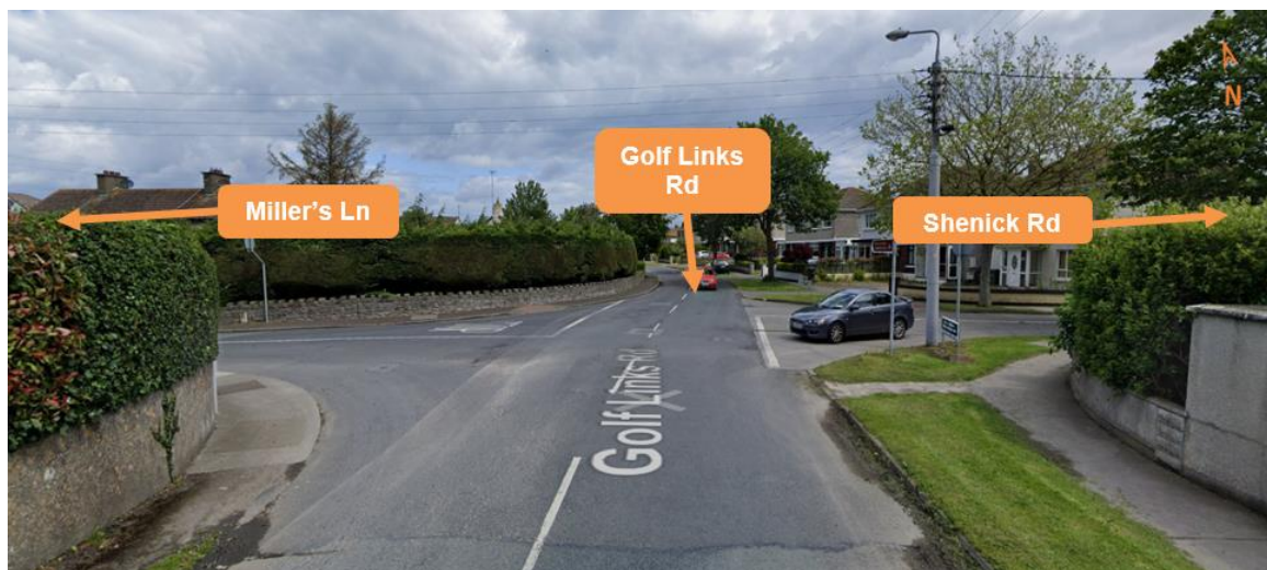
Figure 3.7: Golf Links Rd/Miller's Ln/Shenick Rd Staggered Junction
