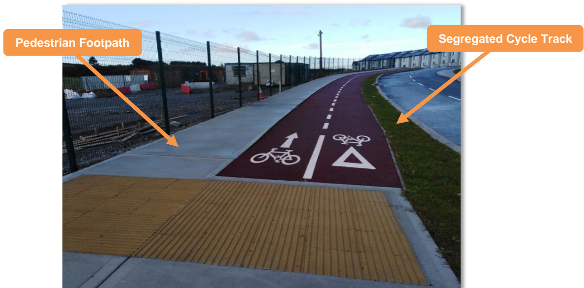
Figure 3.13: Pedestrian and Cycling Facilities At Ballygossan Park Site Access
