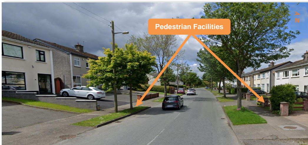
Figure 3.14: Pedestrian Facilities on Miller’s Ln (Towards Skerries Rd/Dublin Rd/Miller’s Ln Roundabout)
